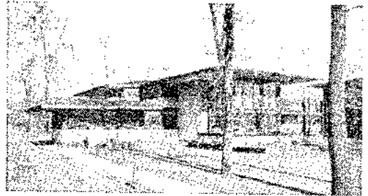
<사진 12> FRANK LLOYD WRIGHT. ISABEL ROBERTS HOUSE. Riva Forest, Illinois, 1907. The slab roof and the low horizontal extension of the wings are interesting. This exterior shows, wright's clarification and purification of standard material.
