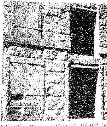
<사진 5> Stone Wall, Union Wharf Warehouse, Boston 1846 The granite posts and lintels for windows and doors were cut in one piece at the Quincy quarries.
