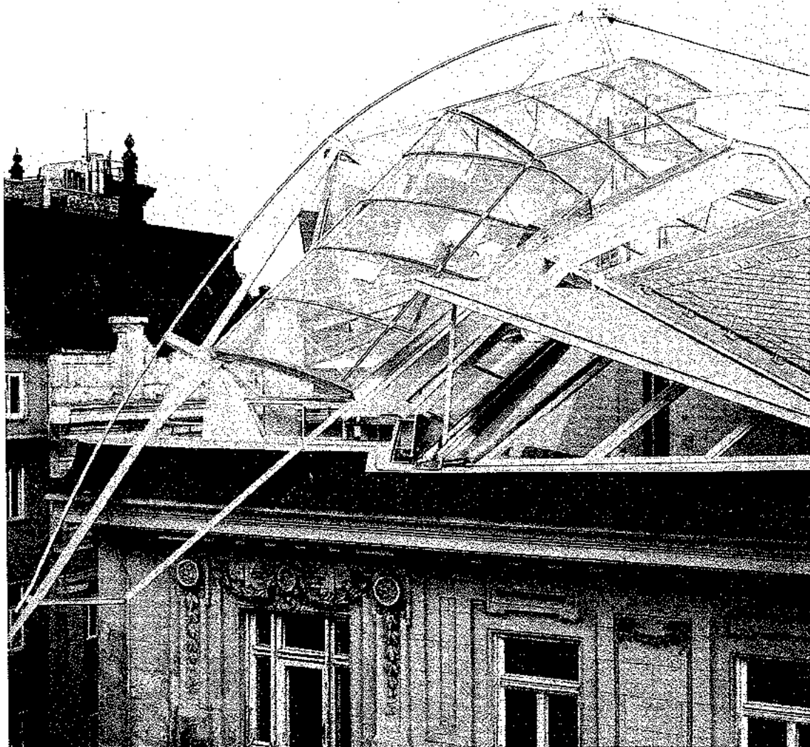
① Rooftop Remodeling 전경(1989)
