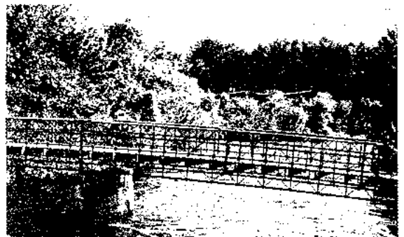
(사진 7) Bridge in Tilton
